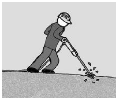
Figure 5. To install a rock anchor, first drill a hole by hand or with a power tool.
